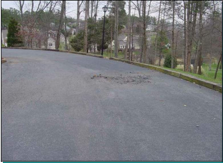
Pavement deterioration
